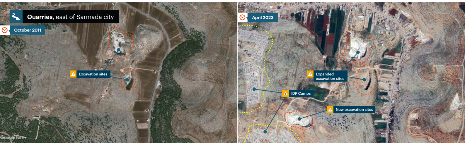
▲ Figure 5. New and expanded quarries east of the city of Sarmadā between 2011 and 2023. These excavation sites are located beside IDP camps that emerged in 2021 and have been growing ever since. Source: Maxar Technologies through Google Earth.
