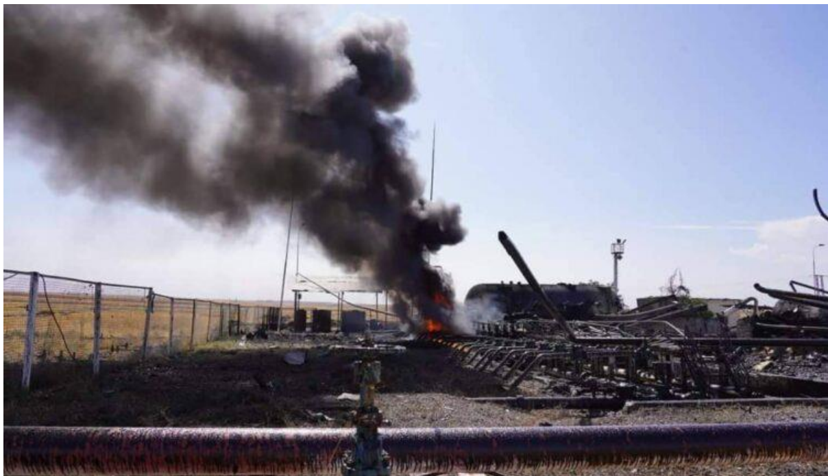
Image 5-Damage at the Suwaydiyah facilities in the countryside of al-Malikiyah/Dêrik city due to the Turkish strike on 5 October 2023. Source: North Press Agency .
