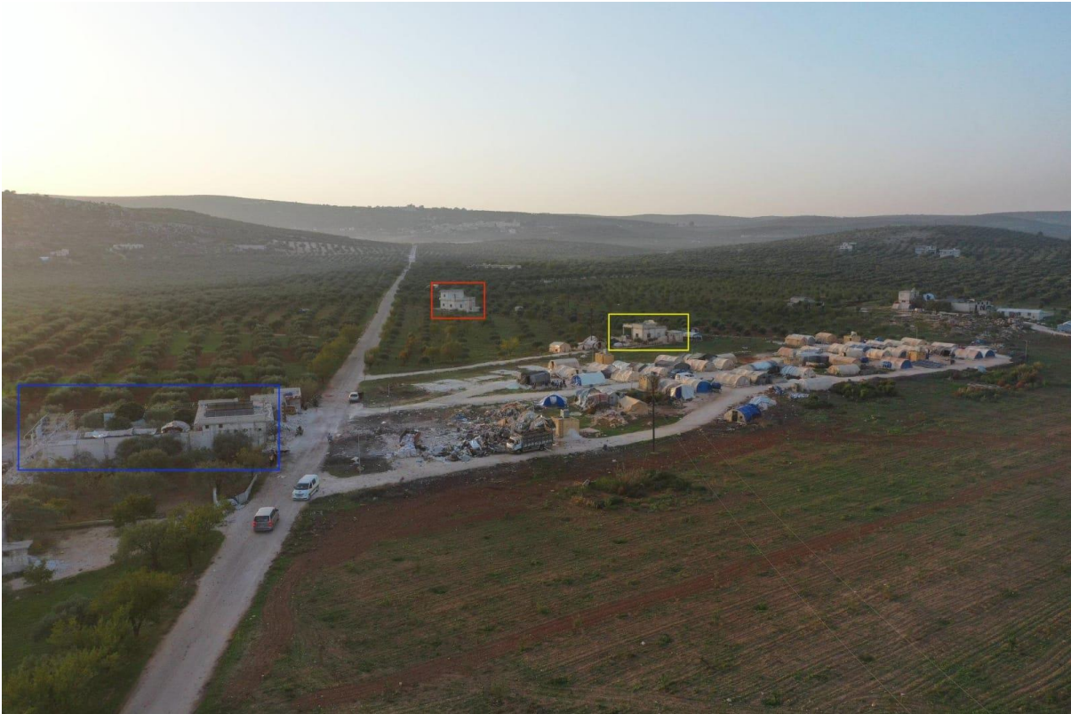
Image 2- A side of the damage caused to Ahl Saraqib Camp by the 24 October attacks. Credit: Syria Civil Defence (The White Helmets) .
