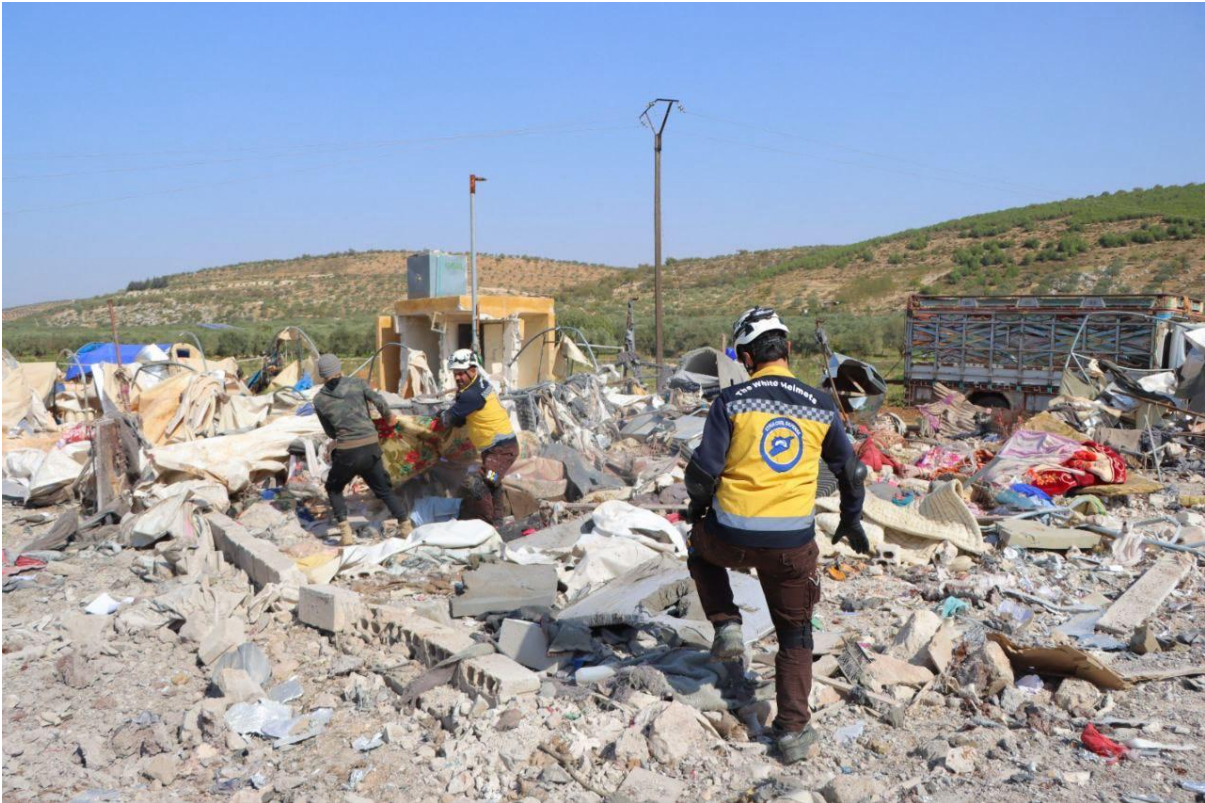
Image 4- A side of the damage caused to Ahl Saraqib Camp by an air strike believed to be Russian on 24 October 2023. Credit: Syria Civil Defence's Telegram channel .
