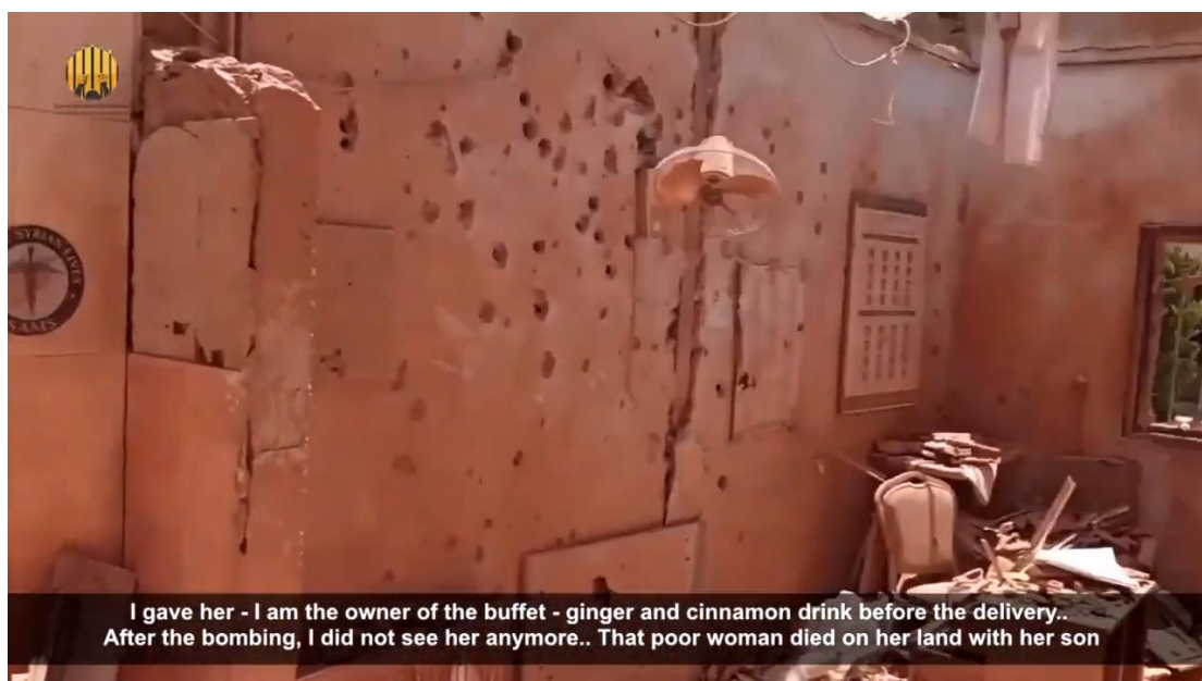
Image 33 - An image displaying damage to the interior. Shrapnel punctured the wall below and to the east of the site of impact. Credit: The National Commission for the Defense of Detainees and Human Rights
