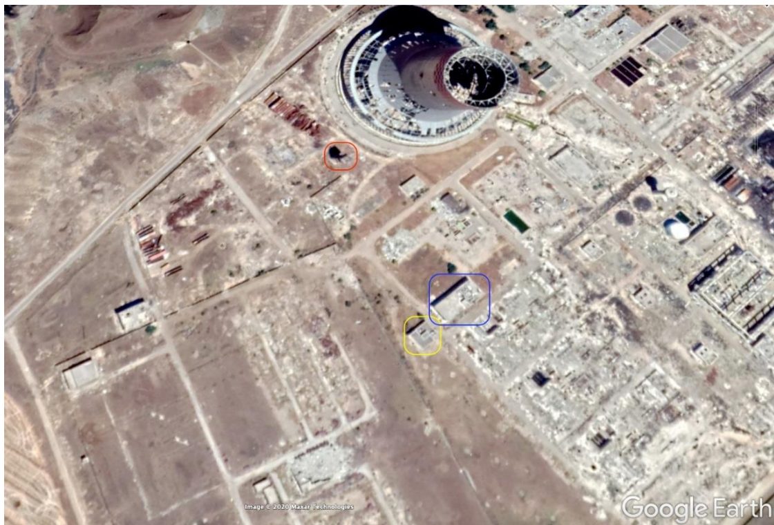
Images 13&14- Analysis of visual evidence of the incident of dropping the Zayzoun power station's cooling tower.
