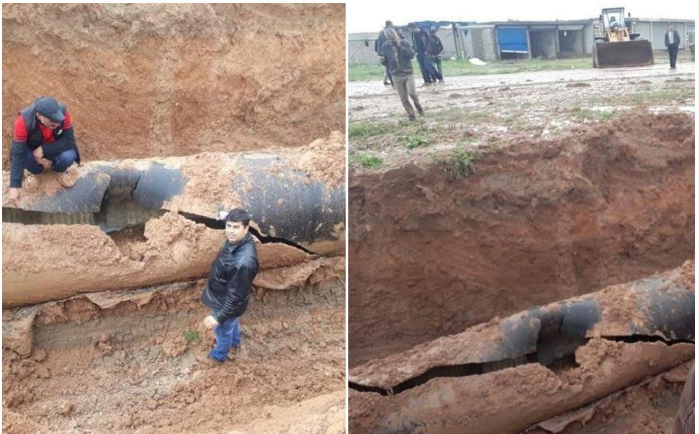
Image (6): Alok pumping station's main water pipe which was put out of service by Turkey and its allies' bombardment with mortars and artillery.
