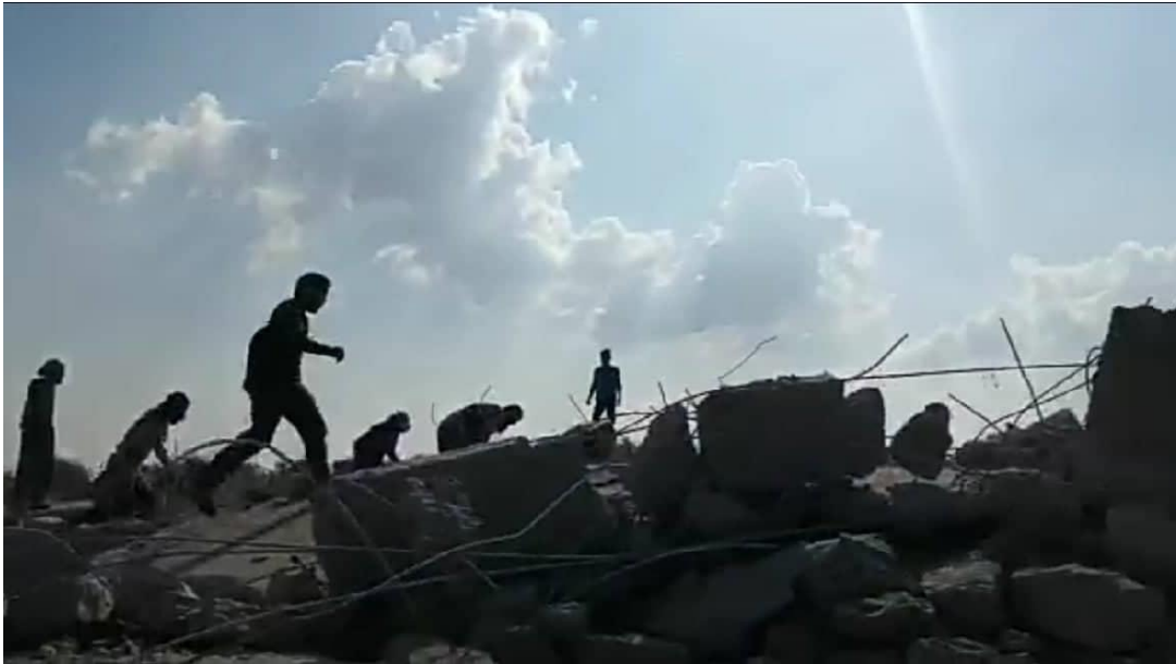
A side of the damage caused to the headquarters of Ansar al-Tawhid group by the attack of August 31, 2019. Photo credit: media activists.
