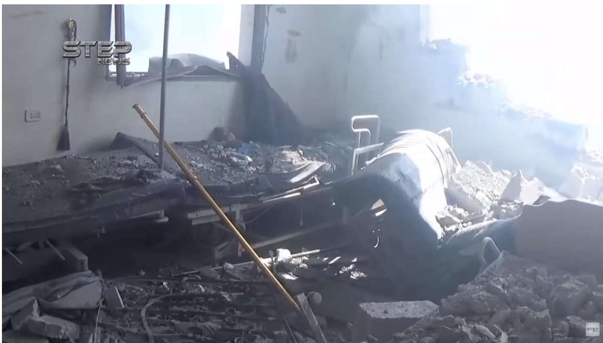
Photo showing the damage in the hospital – Source: Video for “Step” media agency
