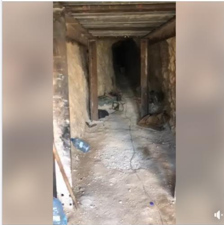
A still taken from the footage published by local activists on August 30, 2018, showing pieces of the railway used to strengthen the tunnel.
