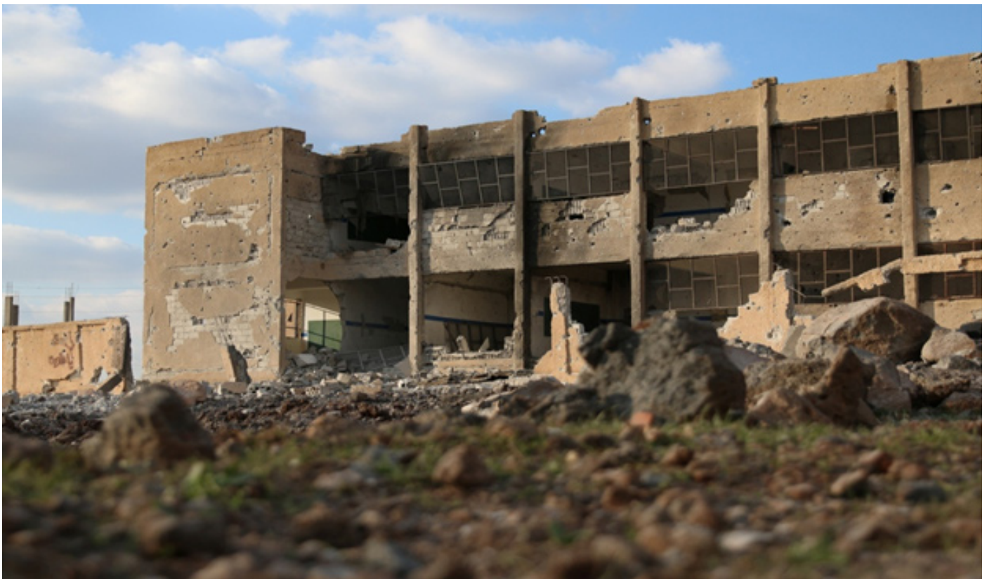
.Image showing damage caused to preparatory school in Busra al-Sham Photo credit: Alaa al-Faqir
