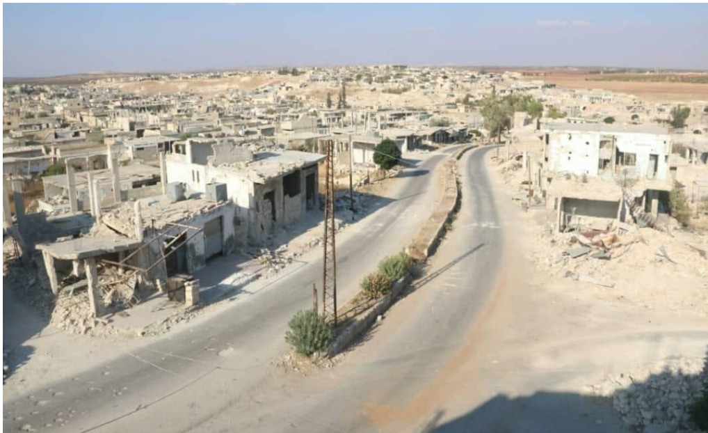
Devastation of civilian houses in al-Lataminah after the attacks of August 2018.
