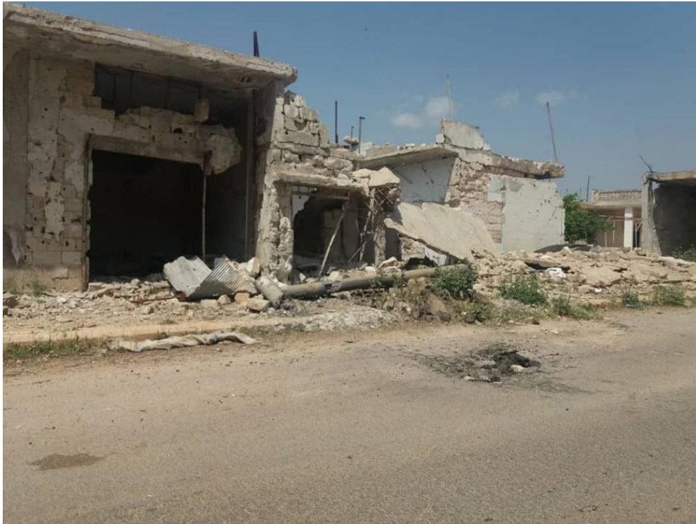
Devastation of civilian houses in al-Lataminah after the attacks of August 2018.
