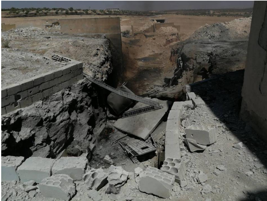
Devastation caused to the Civil Defense Center in al-Tamanah in September 6, 2018 attacks. Photo credit: the Syrian Civil Defense in Idlib province .
