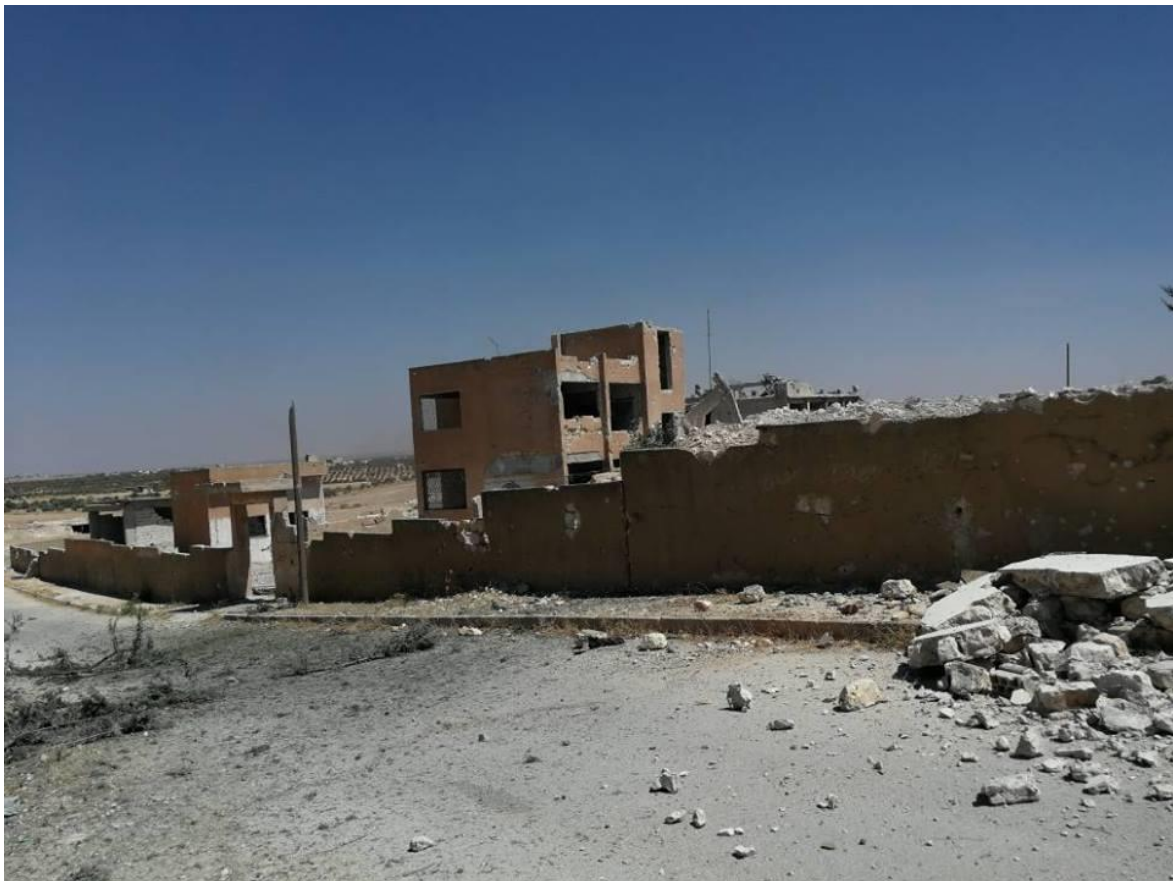
Devastation caused to a primary school in al-Tamanah in September 6, 2018 attacks. Photo credit: The Syrian Civil Defense in Idlib province.
