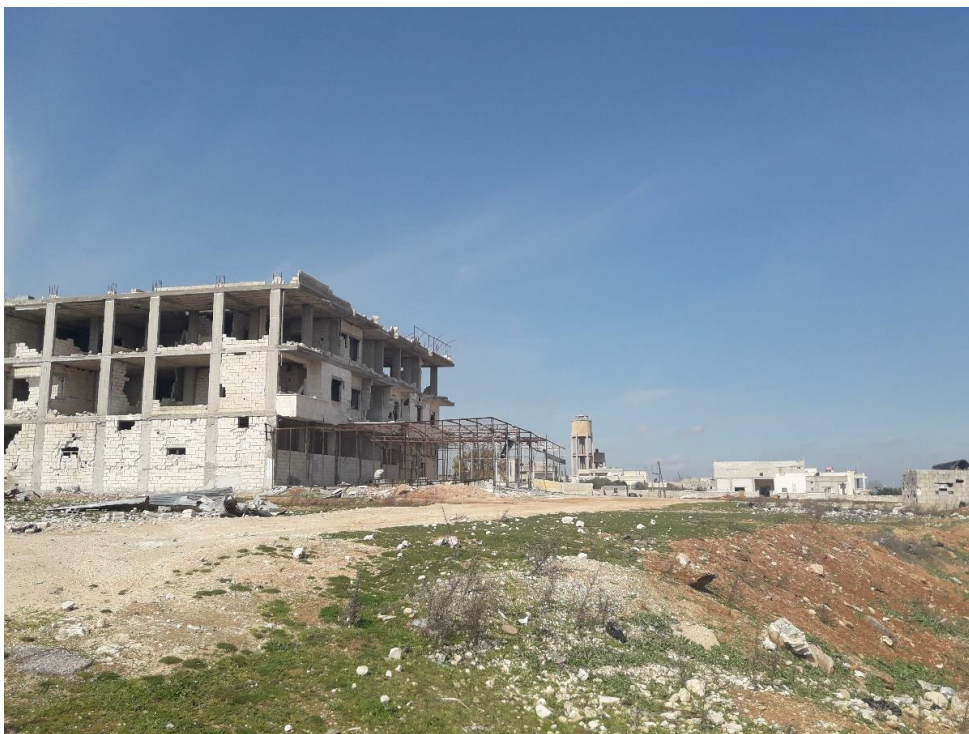
An image shows an aspect of the destruction of the Blood Bank-Thalassemia Treatment Center in Saraqib, following the aerial bombardment of February 5, 2018. Photo credit: STJ
